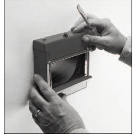
3. Place the FlameStopper Thru-wall Fitting Box over the opening and secure the two bolts.
