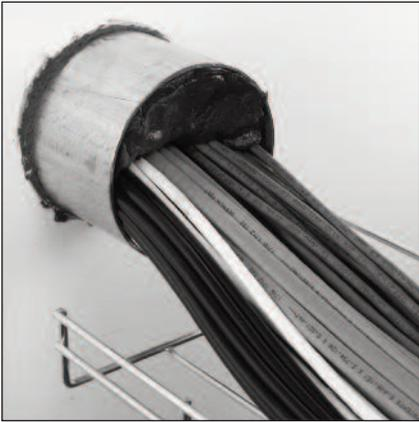
1. Existing conduit with cables. Remove firestop putty.
