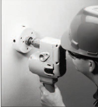
1. Determine location and cut hole in wall using a hole saw, keyhole saw or a core drill.
