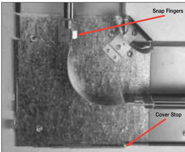
**Step 4.** Install Raceway Covers as shown. Position raceway cover section against cover stop and snap into place.
