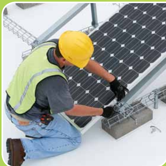
Panels attach quickly and easily with Delta Strut mounting clamps.
