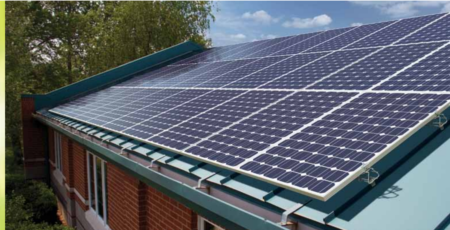
Delta Strut framing attached directly to raised seam roof.
