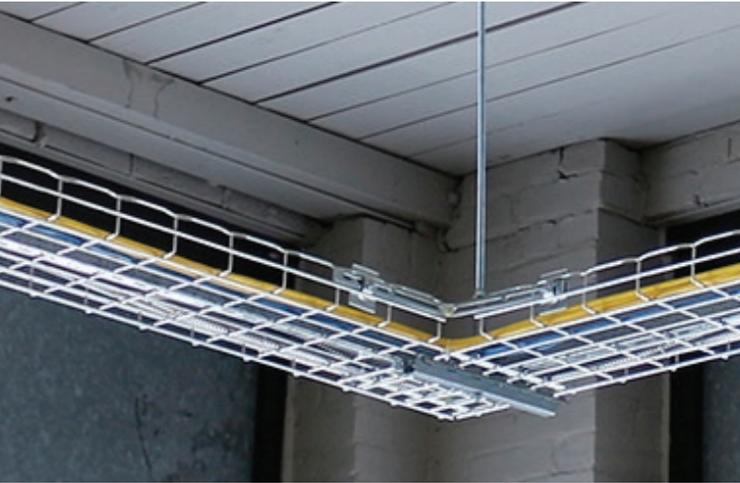
“The tests showed that, in a cable depth of 40 Category 5e or Category 6 cables, there was no identifiable difference in performance between Cablofil cable tray and a perfectly flat surface when tested to TIA/EIA standards.”
