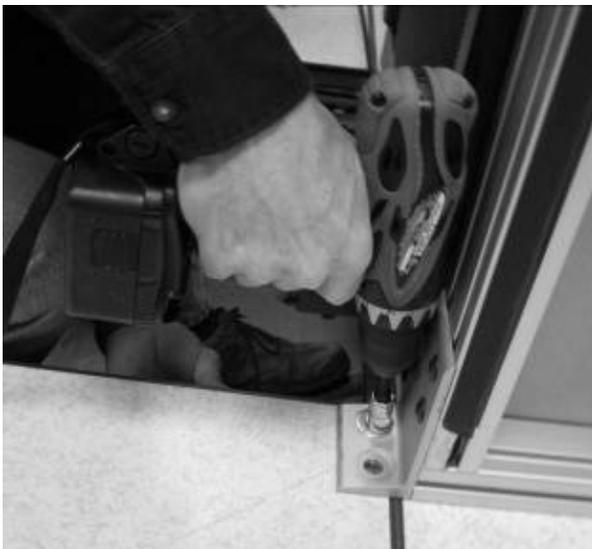
**Step 6:****Attach the doorframe to the floor**
