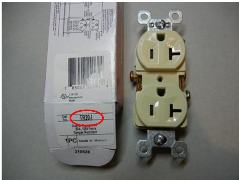
**Front view of recalled receptacle with packaging and model number circled in red**
