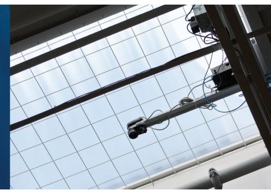
The dual-loop photosensor combines open-loop and closed-loop photosensor technologies to deliver more consistent lighting control and greater energy savings.
