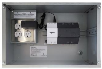
Isolated Class 1 and Class 2 wiring
