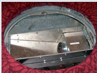
Wiremold/Legrand offers custom services to bring antiquated floor boxes up to date.
