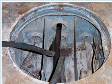
A dated multi-utility floor box damaged by the effects of water entry.
