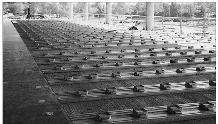
Trenchduct application used as a feeder system for Walkercell Cellular Raceway.
