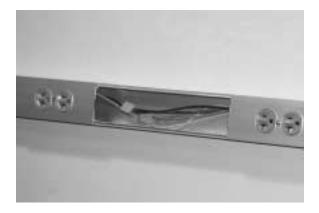
**Step 7** Measure distance between plates and cut necessary covers to match.
