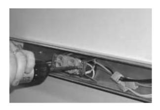
**Step 6** Mount all device plates using provided screws.
