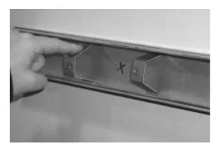
Step 4 Position straps at appropriate mounting distances for the device.
