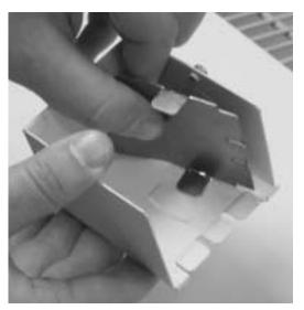
**3.** Attach Entrance End Fitting to the wall using #8 (5/16" [7.9mm] head size) flat head fasteners or equivalent.
