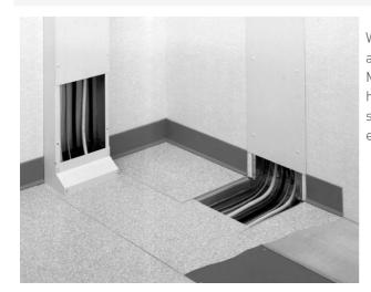
Wallduct is commonly used in the healthcare market to feed wires and cables from electric and communication cabinets to X-ray and MRI equipment. See typical application shown. Because some healthcare equipment requires nonmetallic material in the surrounding area, aluminum Wallduct is used in scan rooms. The equipment and control rooms generally use steel Wallduct.
